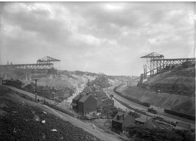
The first Bloomfield Bridge was built in 1914 by the Fort Pitt Bridge Works and was 2,100 feet (640 m) long.
